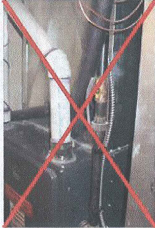
Photo B2 – Armoured cable shall not be in direct contact with copper pipe due to possibility of galvanic corrosion
