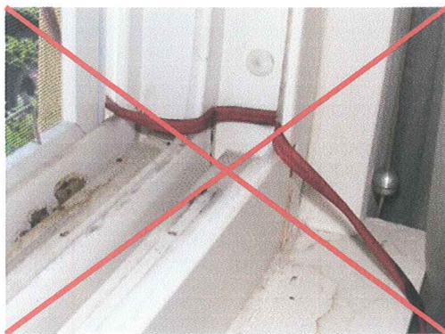
Photo B9 - Cord set stapled to wall or floor
