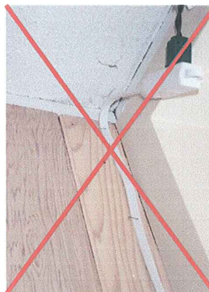
Photo B9 - Cord set stapled to wall or floor
